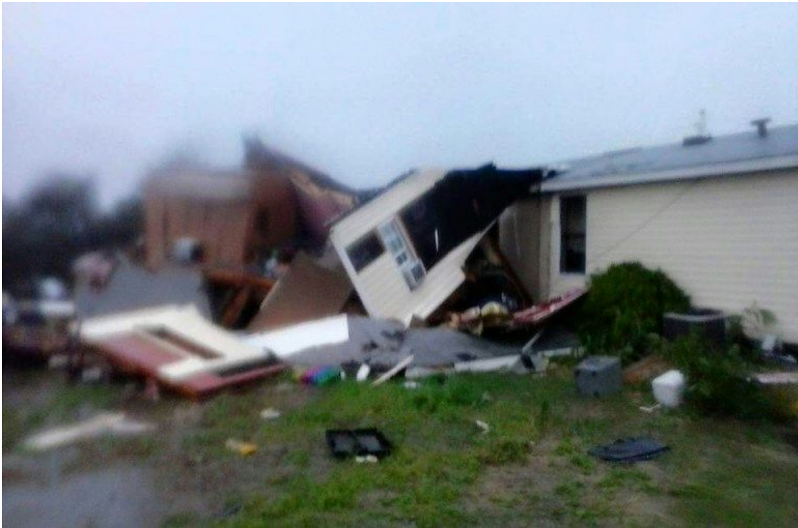
Tornado damage near Pocasset (Grady County).
